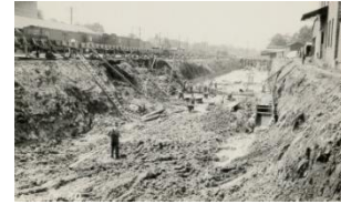
The Channel construction west of N. Academy Street Integral Intercepting Sewer being built at the same time along right side in photograph
