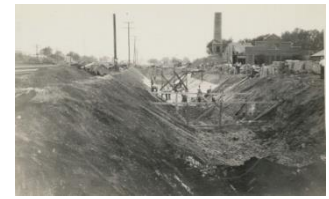
Paving Bricks forming Channel walls
