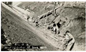
Building the Cedar Fork Creek Channel and laying the Intercepting Sewer pipe
