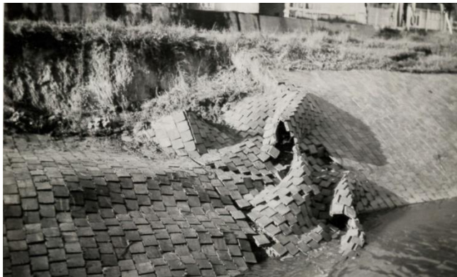
Failure of Channel Paving Bricks
