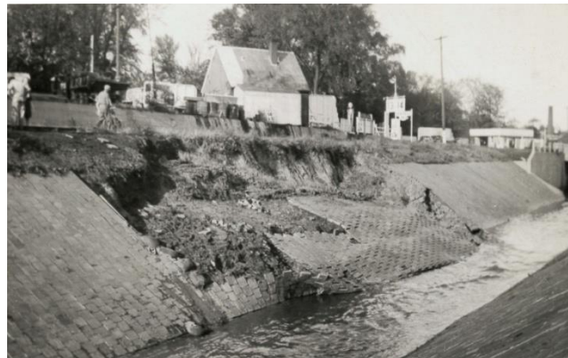
Failure of Channel Paving Bricks
