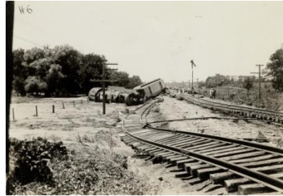
Cedar Creek Flooding washed out rails, causing locomotive derailment
