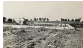
Treatment Plant Trickling Filter and Dosing Tank under construction
