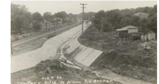
Paving Bricks forming Channel walls looking west from Lincoln Street area
