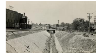
Paving Bricks forming Channel walls looking west from Cedar Street towards West Street
