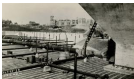
Treatment Plant Trickling Filter and Dosing Tank under construction
